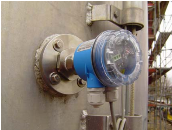
Outdoor installation of FTM20 with polyester housing
